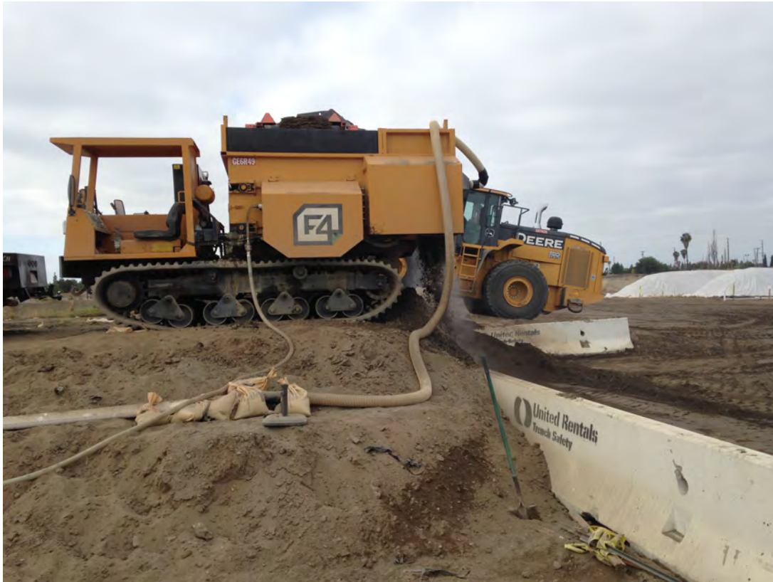
Photo 1: Bulldog Green Remediation, Inc. equipment.
