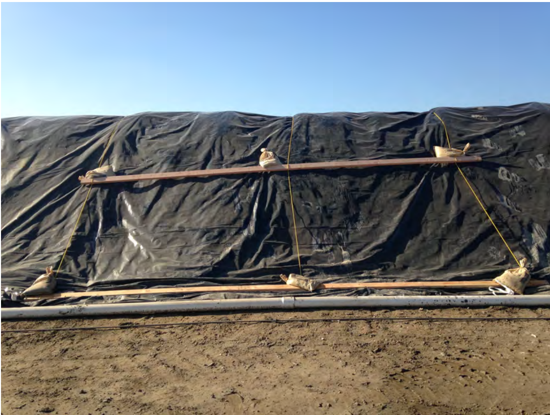
Photo 2: Soil treatment pile cover management.
