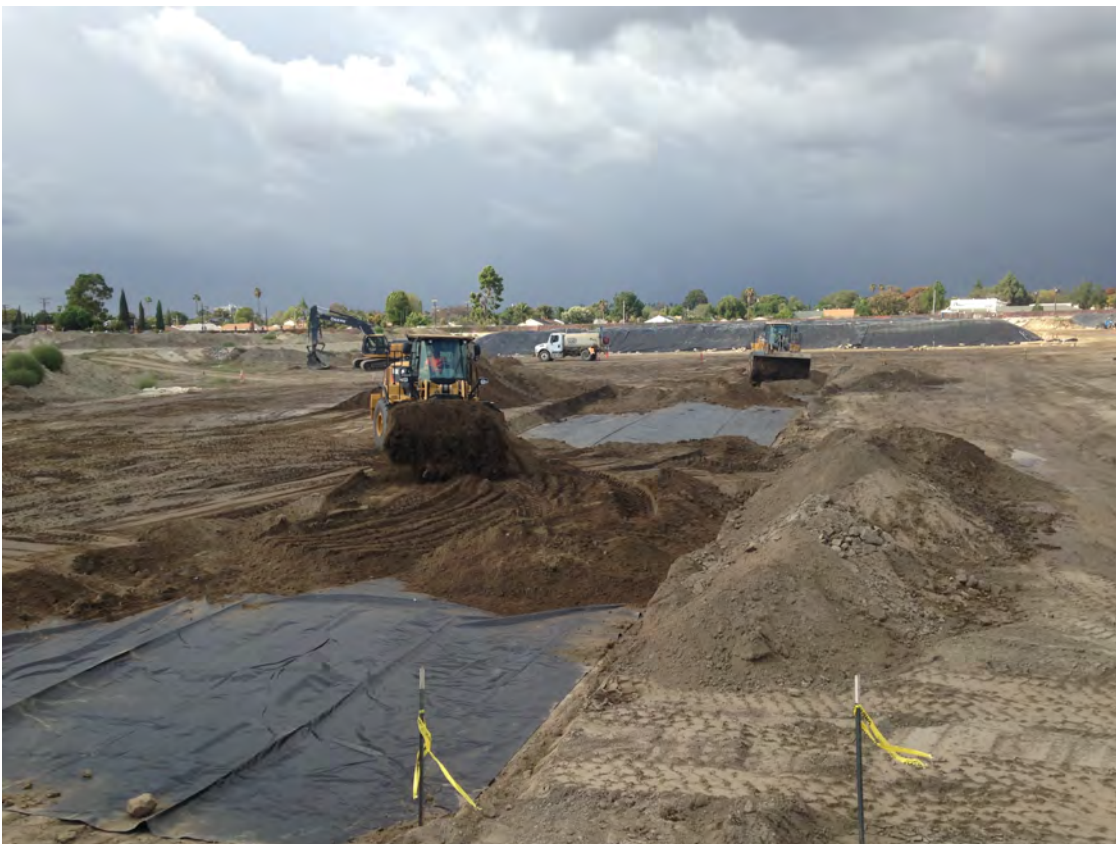
Photo 4: Treatment soil pile construction in former Basin 80013.
