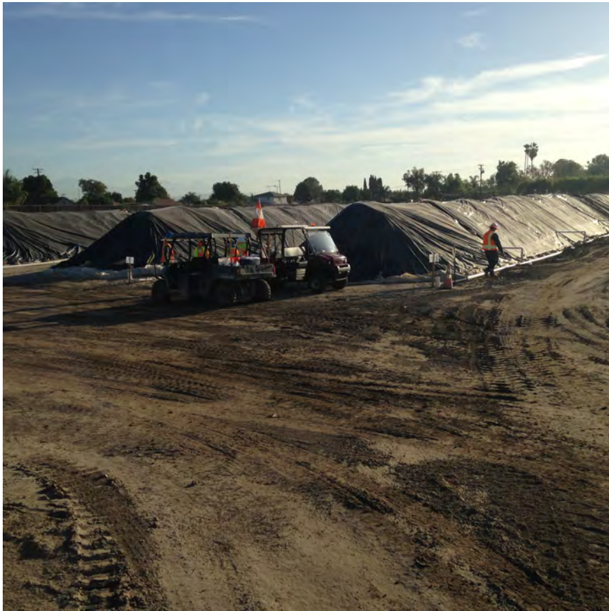
Photo 6: Treatment soil piles.
