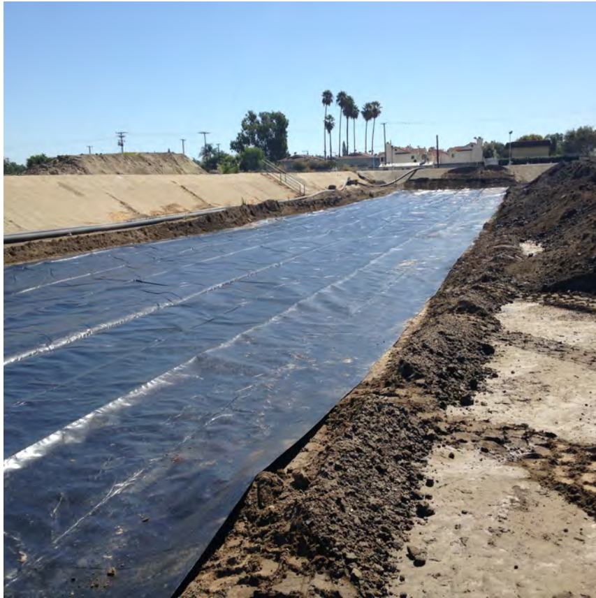
Photo 3: Treatment Soil Pile construction in former Basin 80013.
